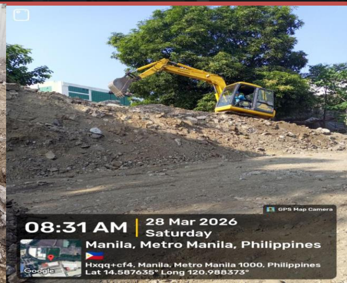
STOCKPILING OF TRANSFERRED SOIL
