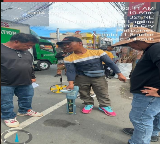
SCANNING THE DEPTH OF THE TAPPED CABLE
