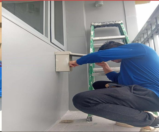
TESTING SND INSTALLATION OF DEVICES
