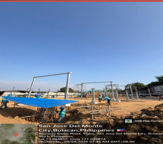
ERECTION OF BUS SUPPORT (BS) STEEL STRUCTURE
