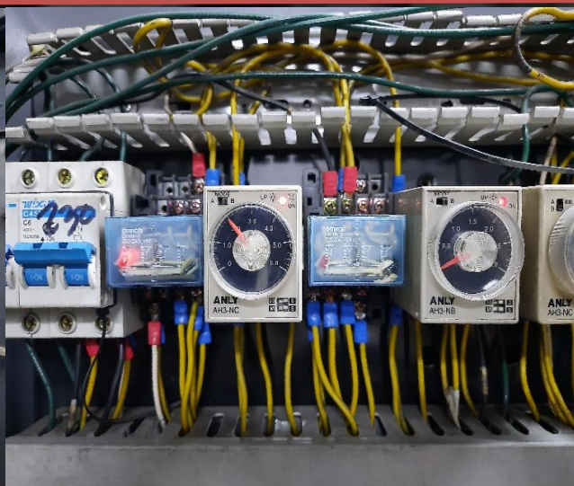
RELAY REPLACEMENT AND SIMULATING THE ATS & GENERATOR ASEANA SNR
