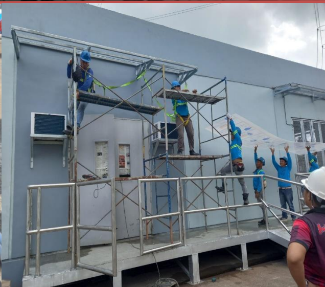
INSTALLATION OF POLYCARBONATE CANOPY ROOFING
