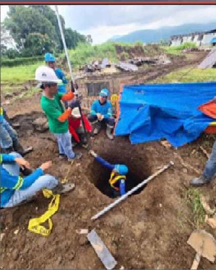
EXCAVATION WORKS FOR BOLBOK
