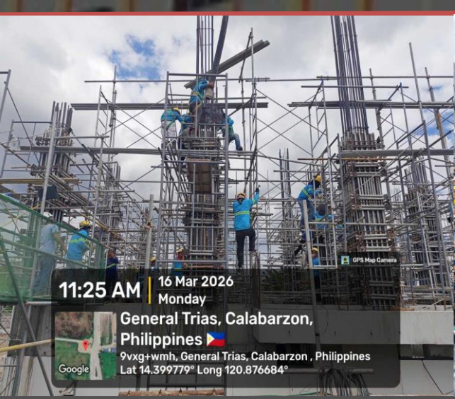
INSTALLATION OF RSB AND FORMS FOR COLUMN 2ND LIFT.
