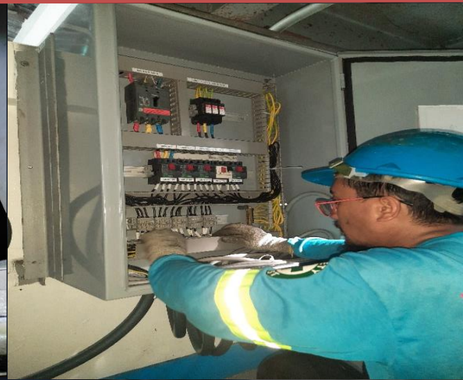
SUPPLY AND INSTALLATION OF MOV CONTROL CABLE @ BALARA PS
