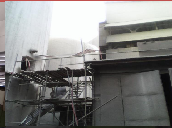
LINE 3 & 4 - CONSTRUCTION POWER (TRANSFORMER & MDP ROOM)
