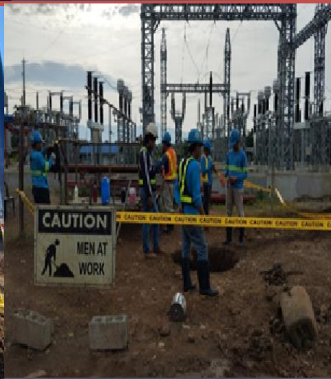
EXCAVATION WORKS FOR LUNTAL
