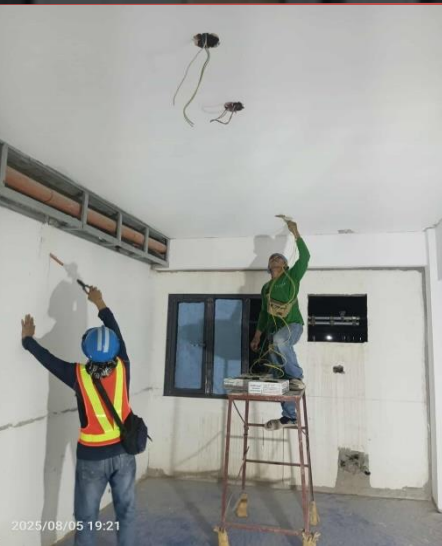
WIRING INSTALLATION @ BUILDING I UNIT FEEDERS
