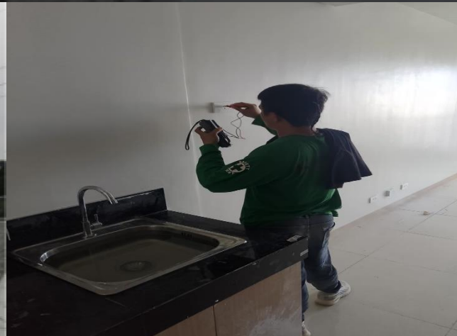
ENGINEERING, PROCUREMENT AND CONSTRUCTION (EPC) OF 69KV POTHEAD AND STEEL STRUCTURES CLIENT: YOKOHAMA TIRE PHILIPPINES, INC. LOCATION: CLARKFIELD, PAMPANGA SCOPE OF WORKS: CIVIL AND ELECTRICAL WORKS
