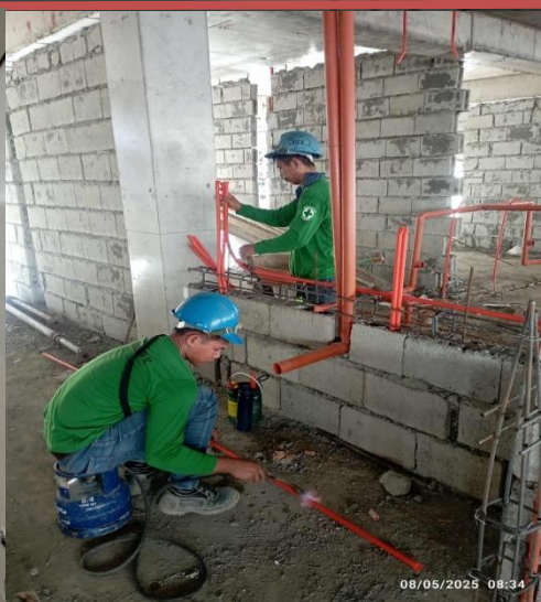
WIRING INSTALLATION @ BUILDING I UNIT FEEDERS
