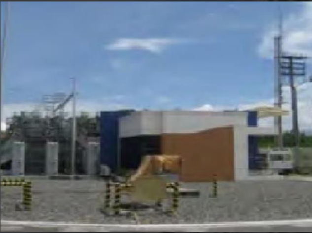
SWITCHBOARD BUILDING EXPANSION 2 x 10 MVA SUBSTATION
