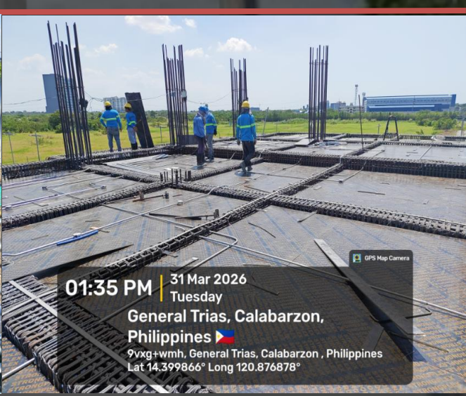
FABRICATION AND INSTALLATION OF FORMS AND RSB FOR 2ND FLOOR BEAMS AND SLAB
