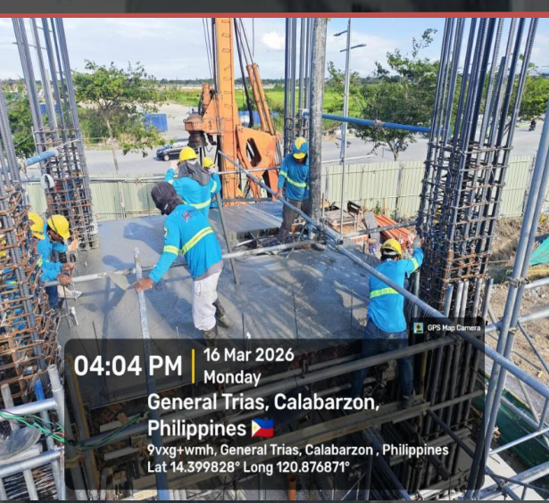
POURING OF CONCRETE FOR GROUND FLOOR COLUMN, MEZZANINE BEAMS AND SLAB
