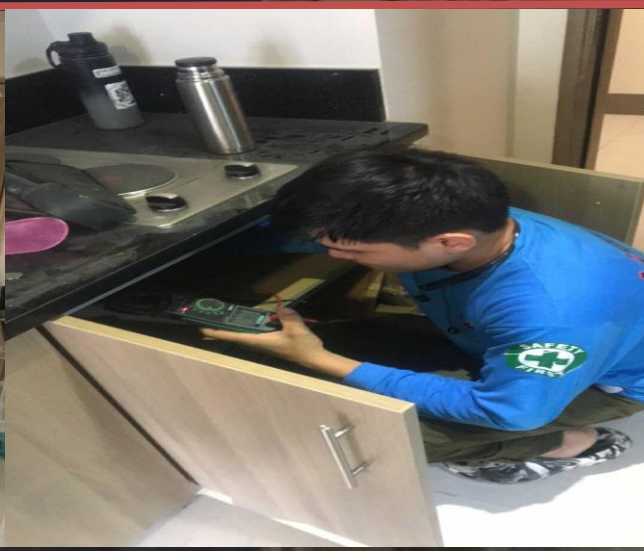
TESTING SND INSTALLATION OF DEVICES
