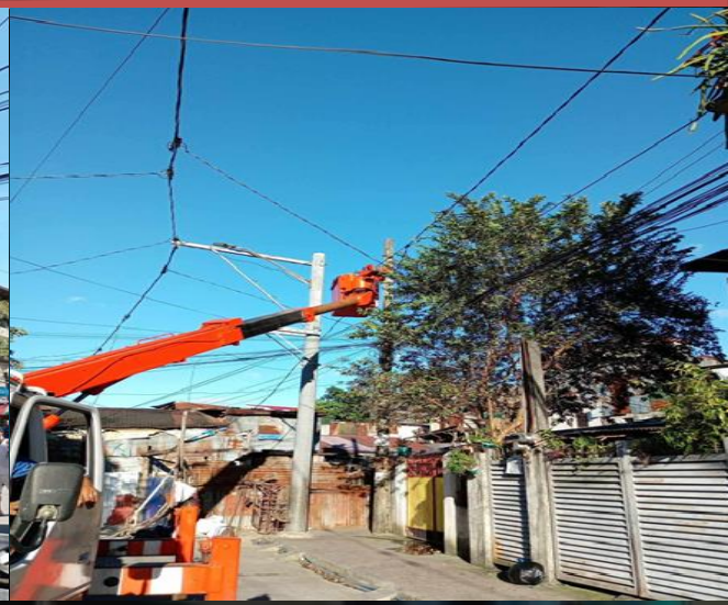
RETIREMENT OF EXISTING SECONDARY WIRES
