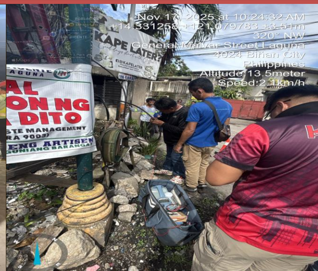
SPLICING THE ENTRY POINT OF THE UG CABLE.
