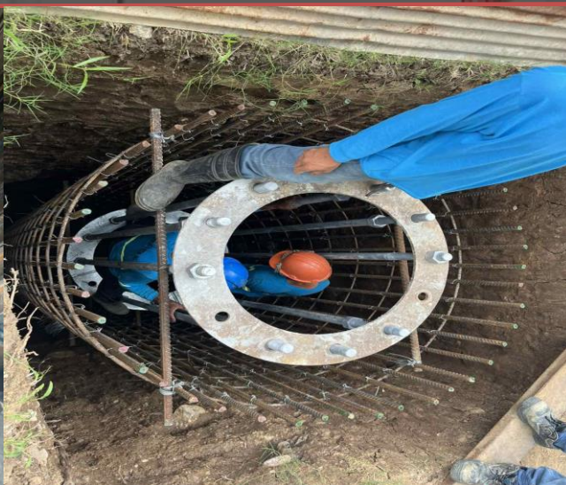
REBAR INSTALLATION OF POLES
