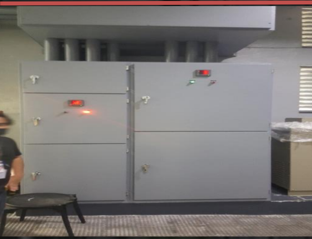
PORSCHE SERVICE LINE UPGRADE & INSTALLATION OF 175KW DC CHARGING STATION
