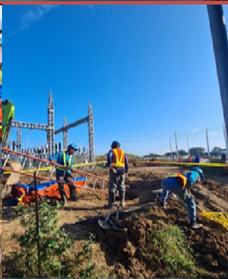
EXCAVATION WORKS FOR LUMBANGAN
