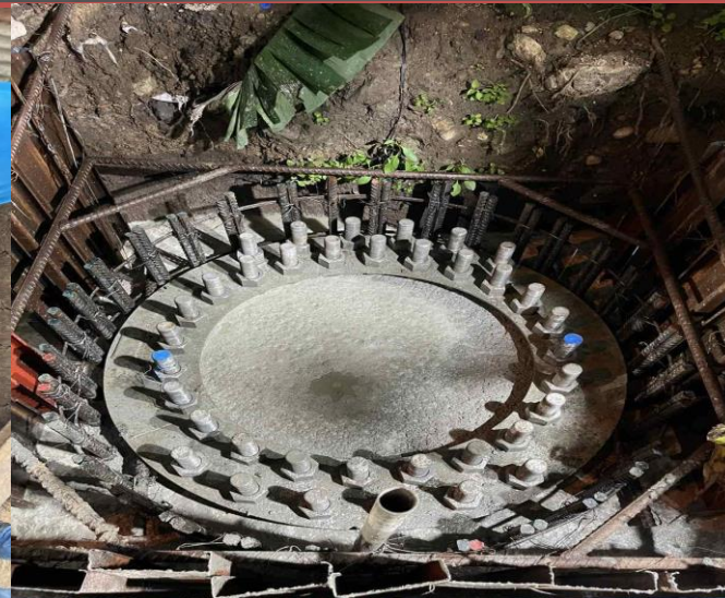
CONCRETE POURING OF POLES
