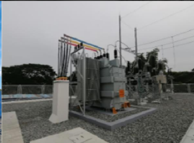
ENGINEERING PROCUREMENT AND CONSTRUCTION (EPC) OF 2X20/25 MVA, 69KV/13.8KV SUBSTATION AND 69KV TRANSMISSION LINE CLIENT: FORMOSA POWER SUPPLY CORPORATION (FPSC) LOCATION: STA. INES, PAMPANGA SCOPE OF WORKS: GENERAL CONSTRUCTION
