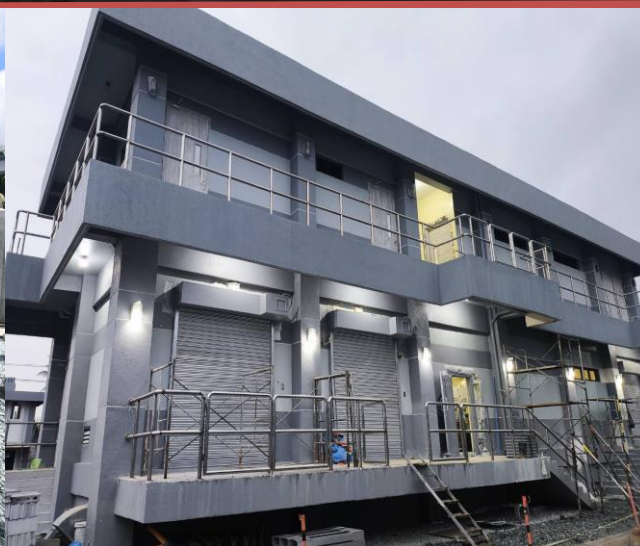
CONTROL BUILDING STATUS
