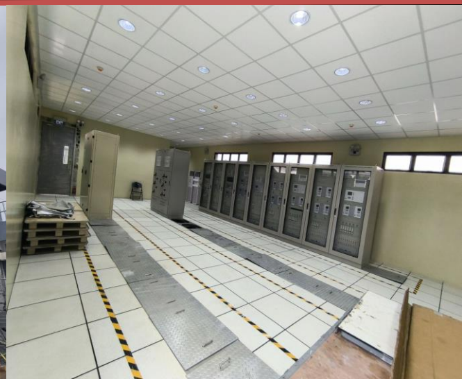
INSTALLATION OF GRATING SUPPORT & COVER @ PXF BANK 1 & 2
