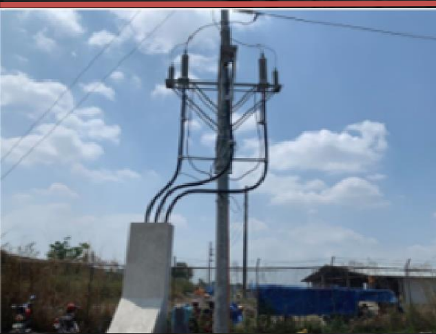
CEDC 69KV UNDERGROUND PROJECT ALONG GIL PUYAT AVENUE CLIENT: CLARK ELECTRIC DISTRIBUTION CORPORATION (CEDC) LOCATION: MABALACAT-ANGELES ROAD, PAMPANGA SCOPE OF WORKS: CIVIL WORKS
