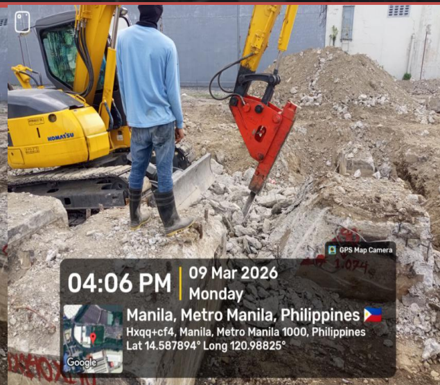
CONCRETE PAD BREAKING
