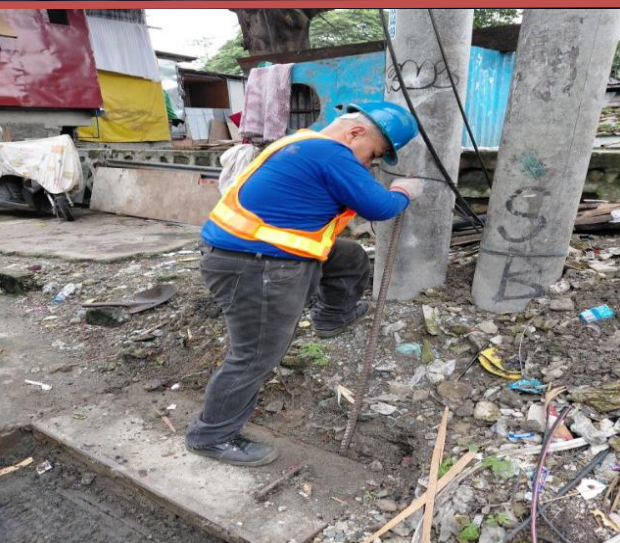
CABLE PULLING AND WIRING @ DAGOHOY LS
