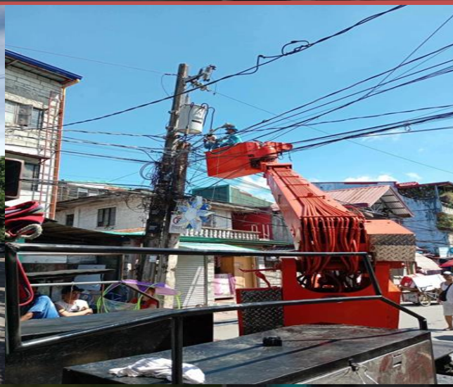
CONNECTING TO TRANSFORMER
