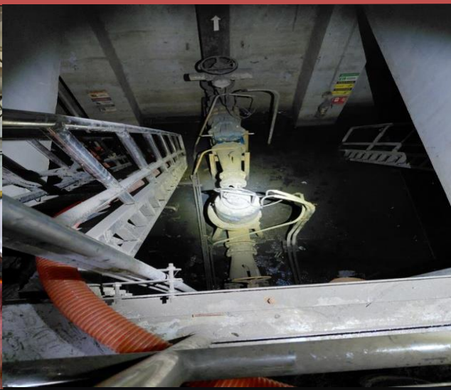
REPAIR OF SEWAGE SUBMERSIBLE PUMP @ MARIKINA NANGKA PS
